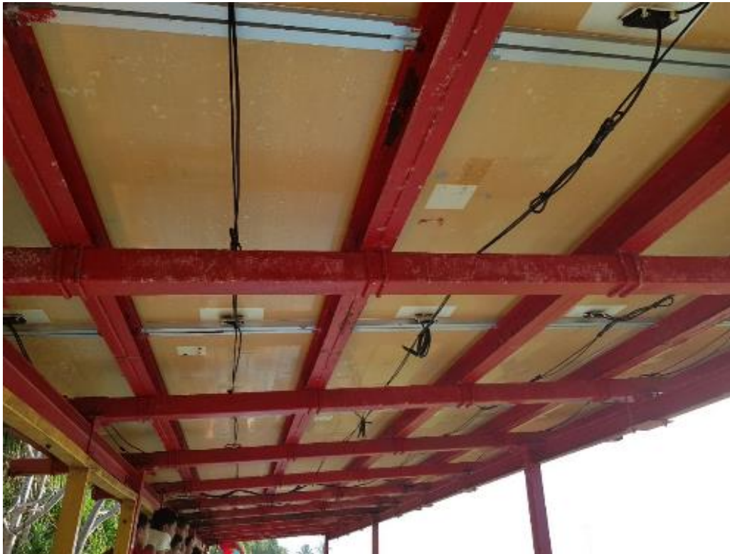
Figure B.32: The grandstand solar project module condition after 11 years of operation. Delamination, discolouring, loose junction boxes and damaged wiring is visible.
