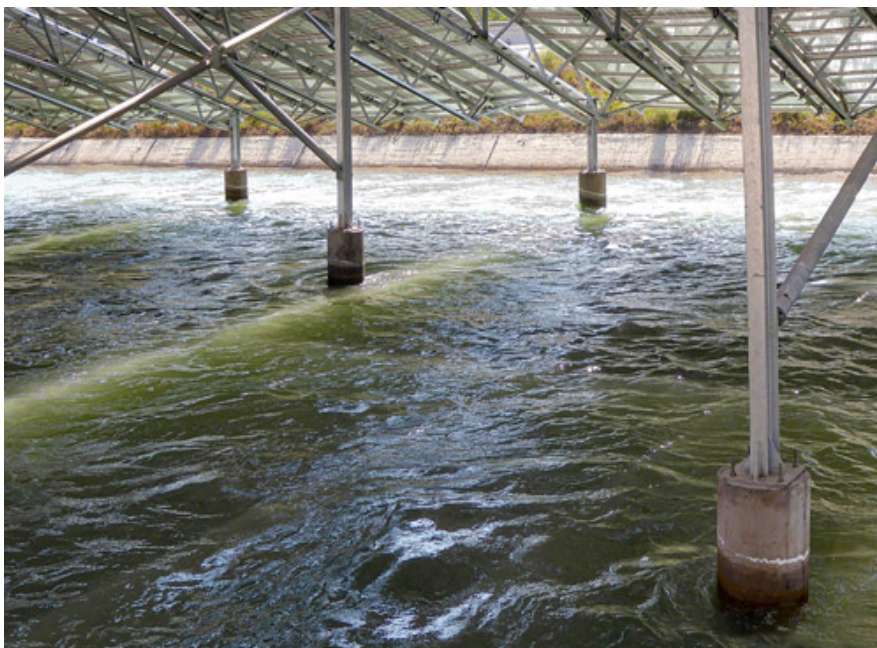
Figure 7.6: P4P Energy's over water raised fixed structure system implemented at scale. 18
